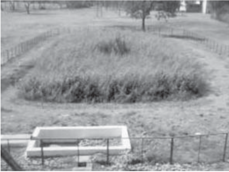
Figure 2 Constructed wetlands at Ravindranagar, Ujjain, Madhya Pradesh
